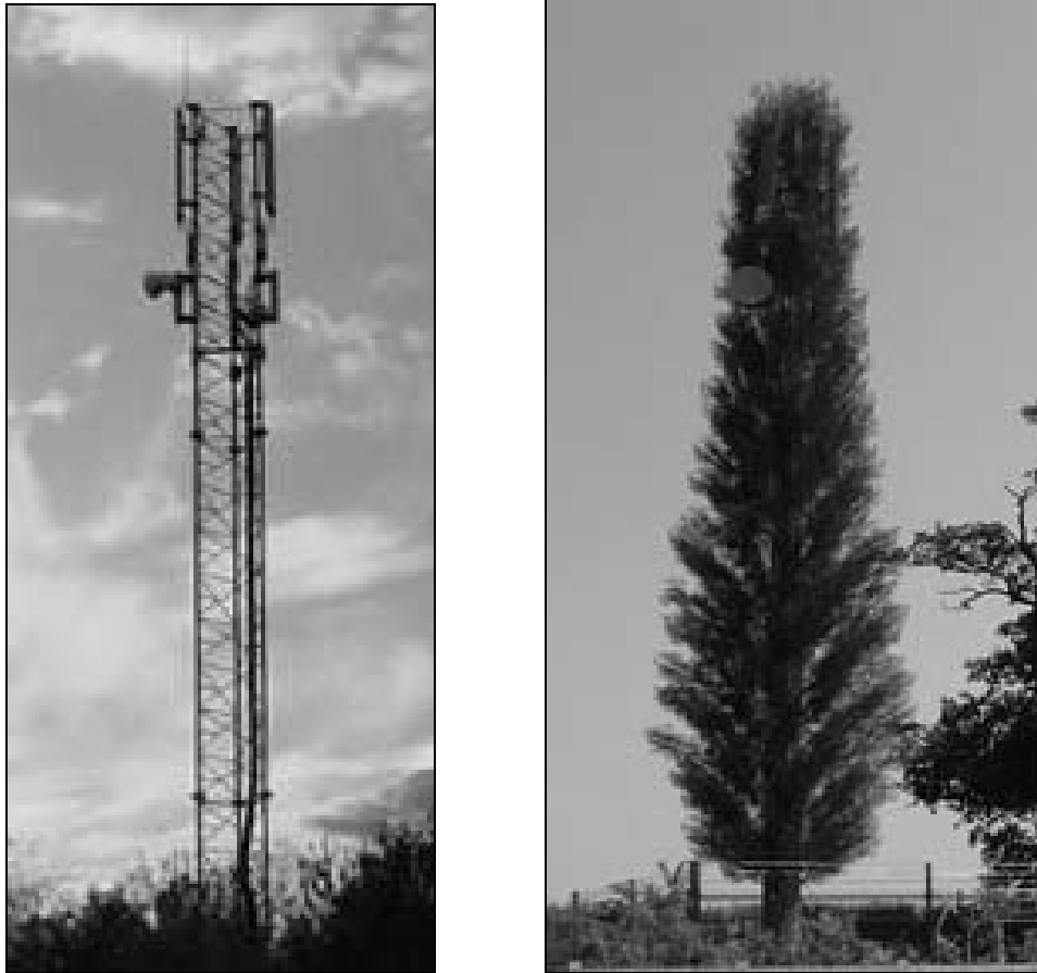
Figure 1a & 1b. Standard mobile phone tower and the FLI Cypress tree tower
