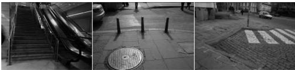
Figure 1. Images of a few examples of non-compliance with regulations. Photo 1. Lack of elevator or platform at the exit of the newly built subway station Sofia University "St. Kl. Ohridski" by the side of the King's Garden; Photo 2. Lack of tactile ground and insufficient space for crossing on Blvd. "Vitosha"; Photo 3. Crosswalk ending with high curb at one of the entrances of the church "St. Al. Nevsky"
